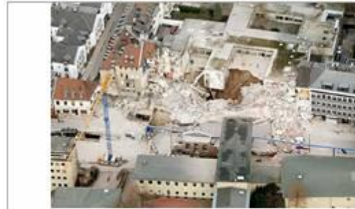
Fig. 4. Aerial view, 2009 collapse of Cologne's Historical Archive, due tunnel construction.
