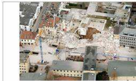
Fig. 4. Aerial view, 2009 collapse of Cologne's Historical Archive, due tunnel construction.
